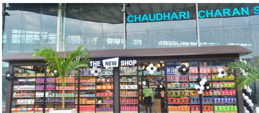
Landside, Chaudhary Charan Singh Airport, Lucknow
